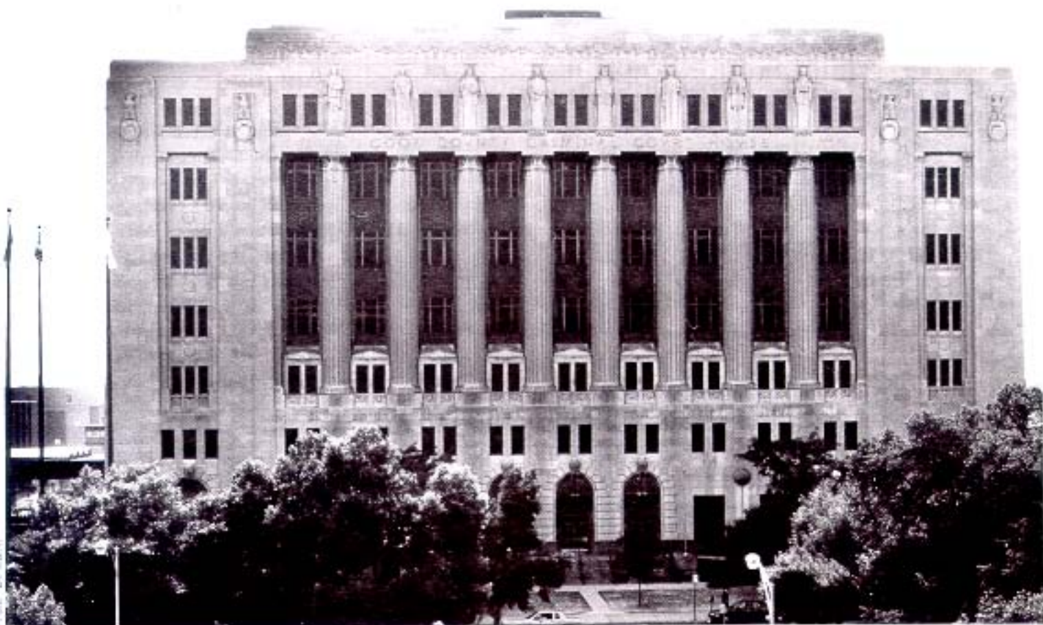
The Cook County Criminal Court building at 26th Street and California Avenue in Chicago houses the nation's largest felony trial-court system under one roof.
